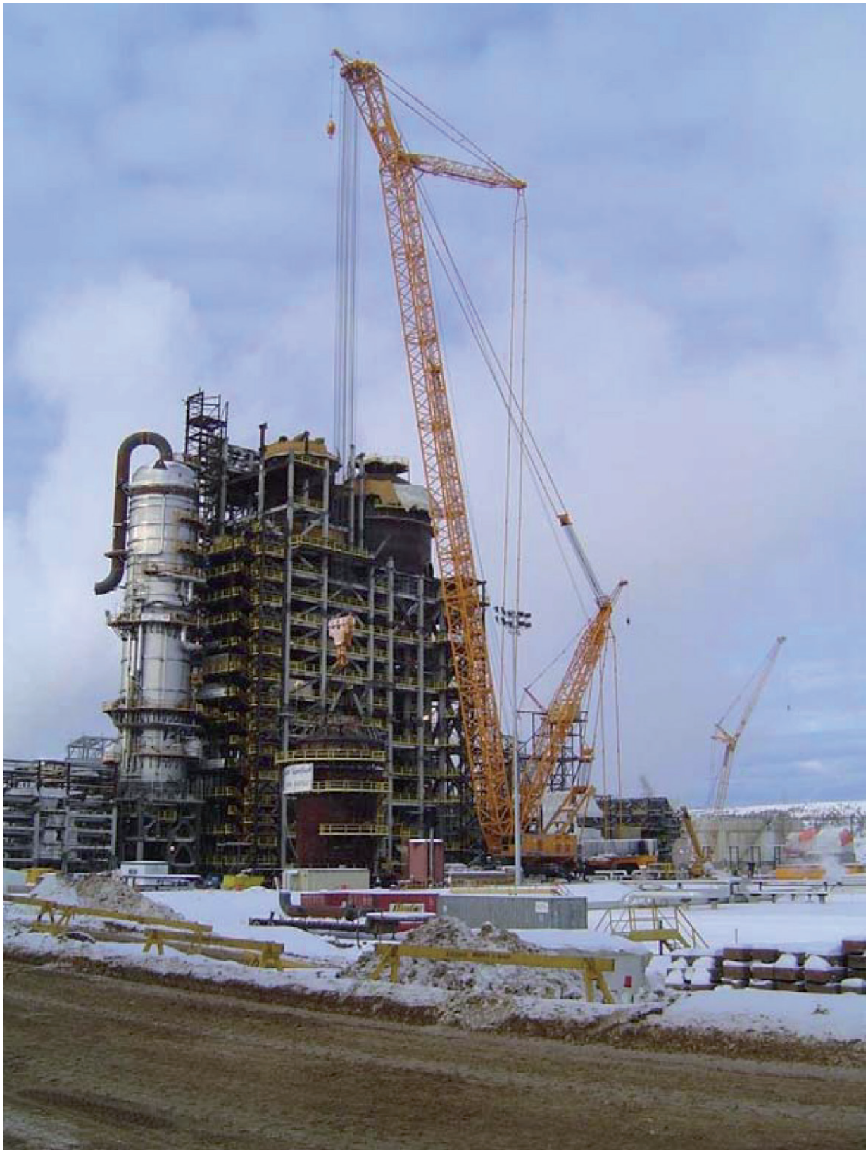
Fig. 13: Terex-Demag CC 8800 Mobile crane involved in lifting work at a chemical refinery. (Photo courtesy Hans-Peter Franzen, Terex-Demag).
